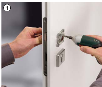
1 Place the base and tighten the screws
