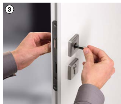
3 Insert the solid profile spindle
