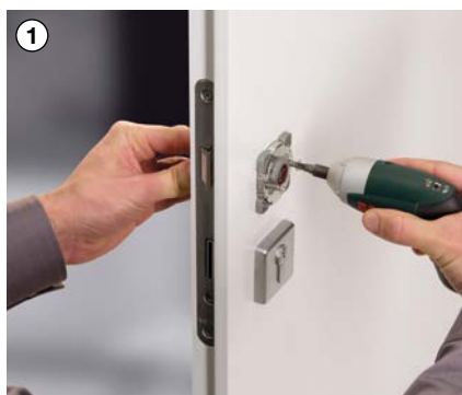
1 Place the base and tighten the screws
