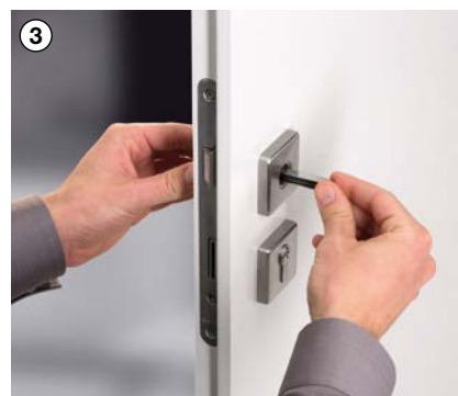
3 Insert the solid profile spindle
